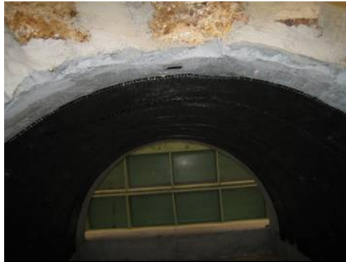
Figure 14. Disposition des renforts
